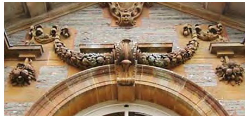
Figure 46: Hestercombe, Somerset. Garland and keystone on Lutyens designed Orangery.
