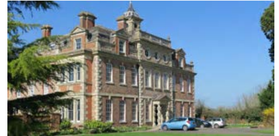
Figure 73: Walsworth Hall, Gloucestershire. Three circular windows in the attic.
