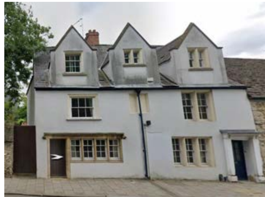
Figure 63: Vernacular houses, St Giles Street, Oxford. Stone faced (and rendered) dormers.
