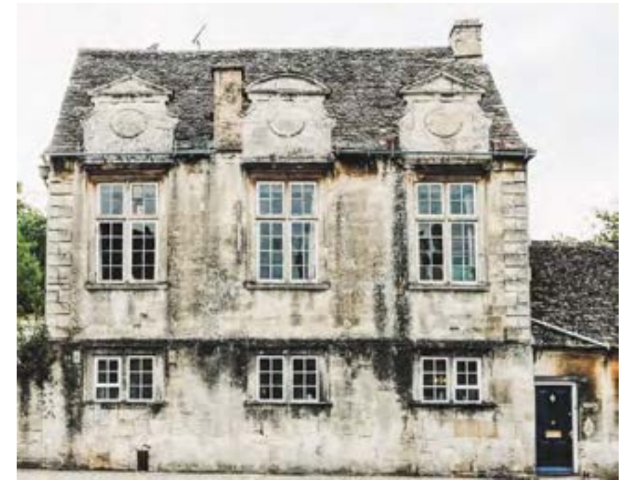
Figure 64: Cobb House, Burford, Oxfordshire. The shaped gables add emphasis to the windows below. It is not difficult to imagine attic windows in the blind ovals.
