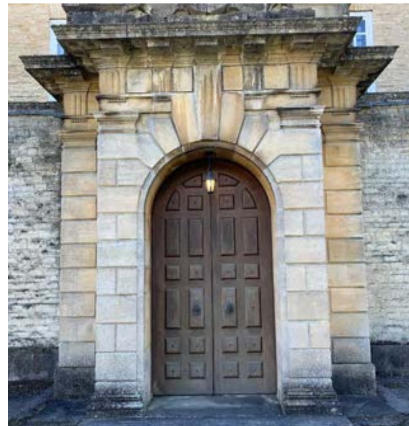
Figure 37: Main entrance to Middleton Park, Oxfordshire. Lutyens plays Mannerist/Baroque games with rustication.
