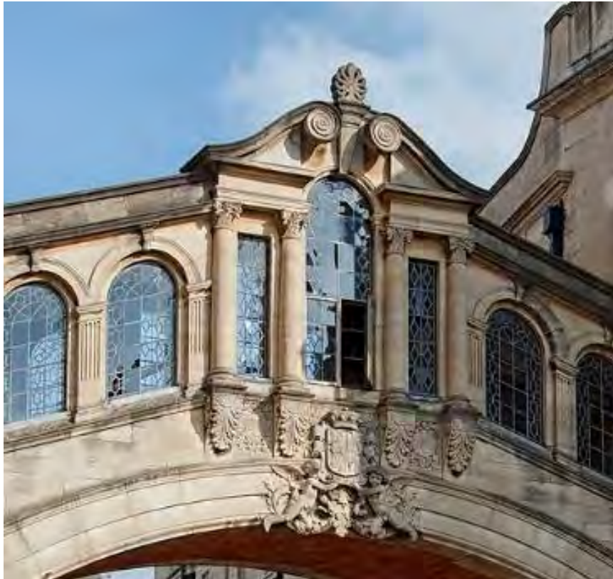
Figure 19: The "Bridge of Sighs", Hertford College. The design is more like a Baroque reimagining of the Rialto bridge.
