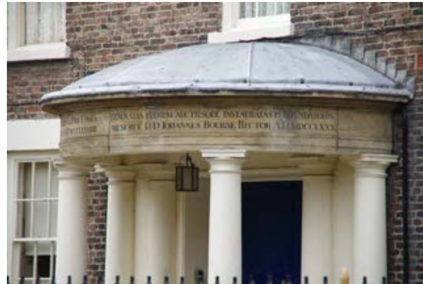
Figure 44: Detail of the Charter House porch showing the lead covered dome.
