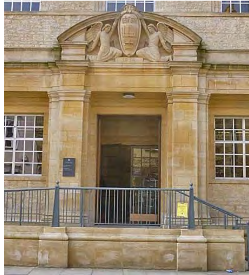
Figure 24: The New Bodlian Library, Oxford. Aside from the broken pediment with its escutcheon and angels, Giles Gilbert Scott plays Baroque games with superimposed layers of pilasters.
