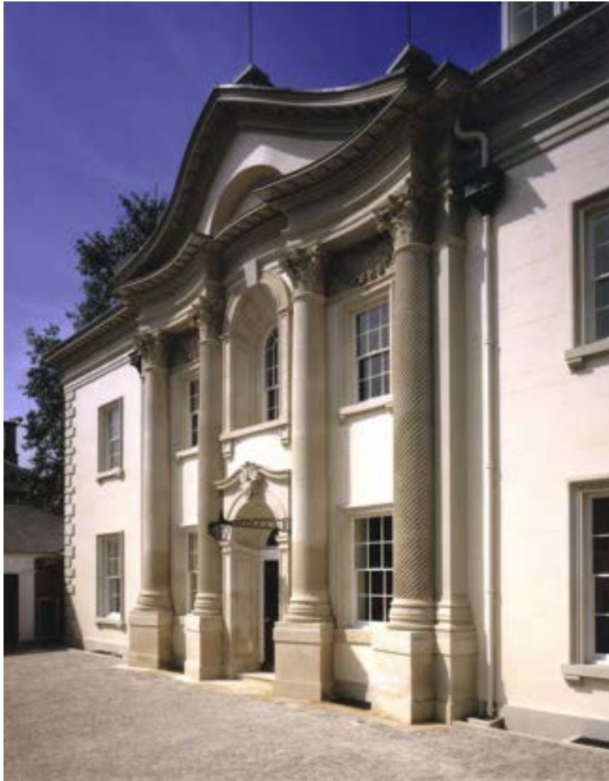
Figure 91: The Corinthian Villa, Regent's Park. The first serpentine façade built in England.
