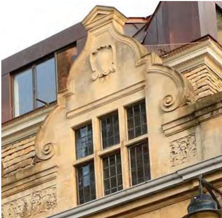
Figure 66: Detail of the Rhodes Building, Oriel College, Oxford. Champneys seem to have adapted the shaped gables from the old quad as dormers for his new building.
