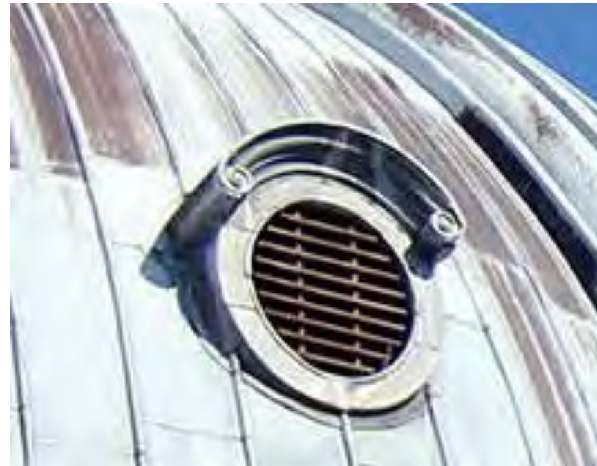
Figure 68: Ventilator, Radcliffe Camera, Oxford. A small cornice gives architectural presence to a simple feature.
