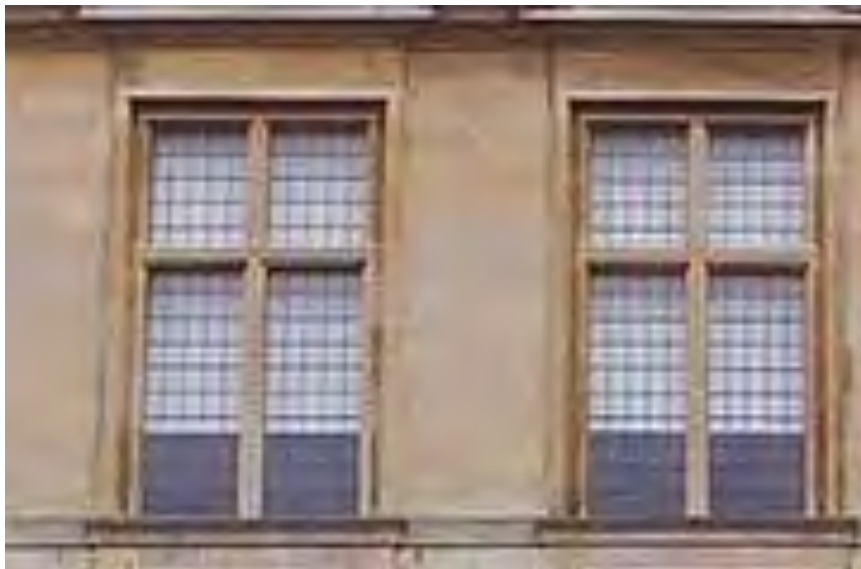
Figure 61: Casement windows, The Old Ashmolean, Oxford. The limitations of seventeenth century glass making meant that many small glass quarries had to be leaded together to form a single sheet.
