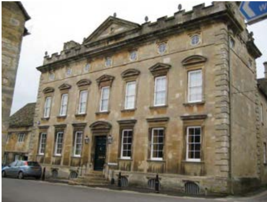
Figure 26: The Great House, Burford. The classical language of the lower stories is fairly conventional, the attic storey and crenelated parapet are much less conventional.
