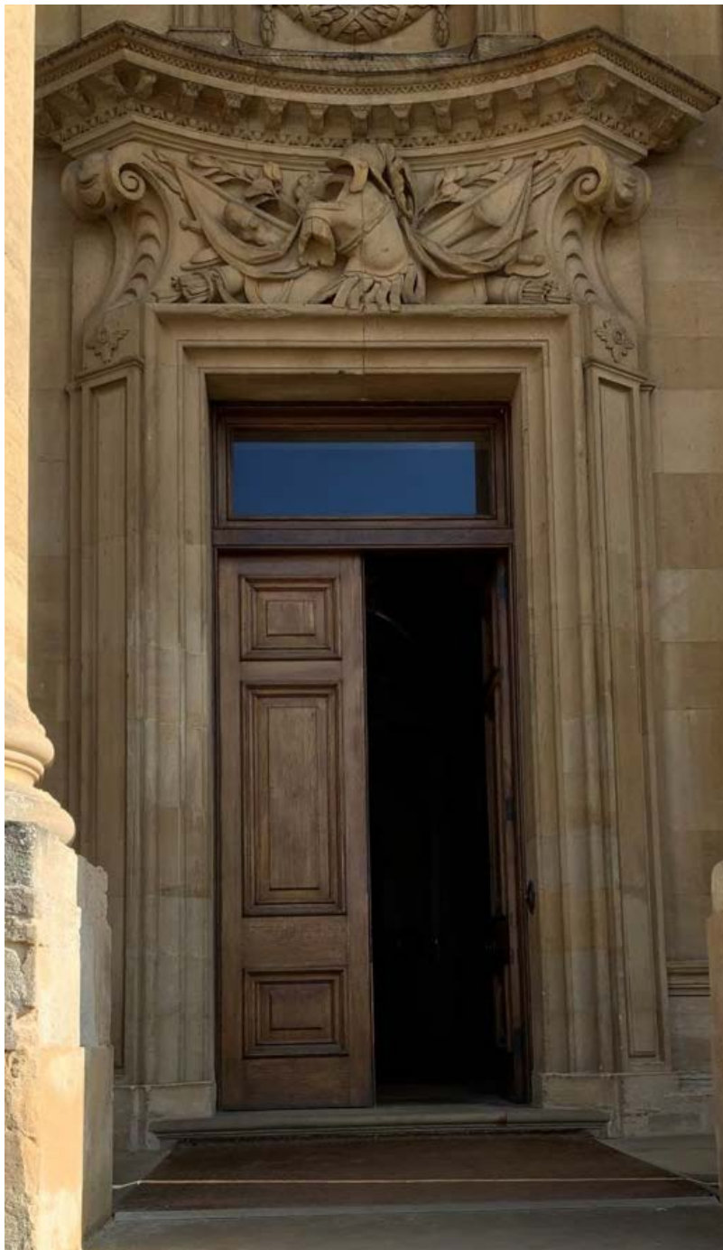
Figure 30: Door at Heythrop House, with a Borromini style concave cornice.
