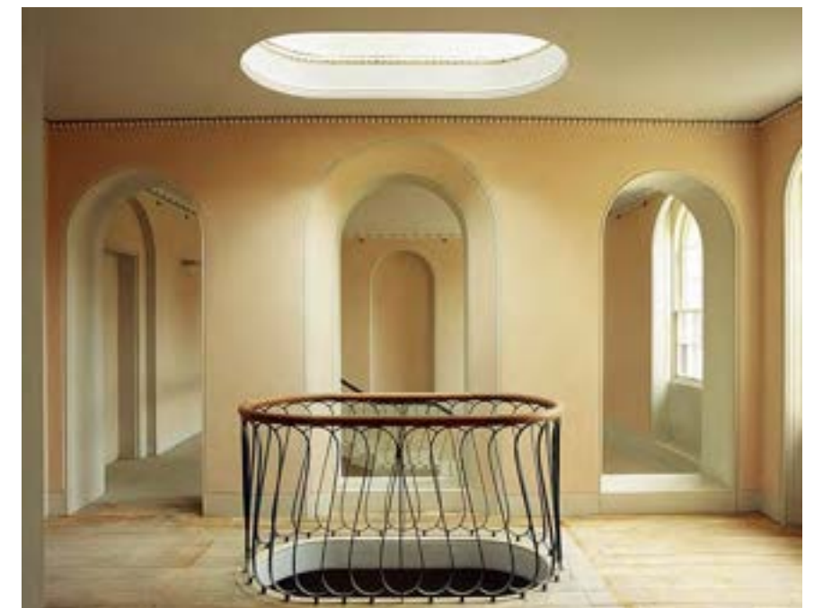
Figure 95: The tribune, Moggerhanger. An oval lightwell with a skylight over.
